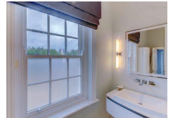
Half obscured glass and bottom sash horns
